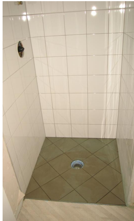
10. Tiling floor then grouting & silconing.
