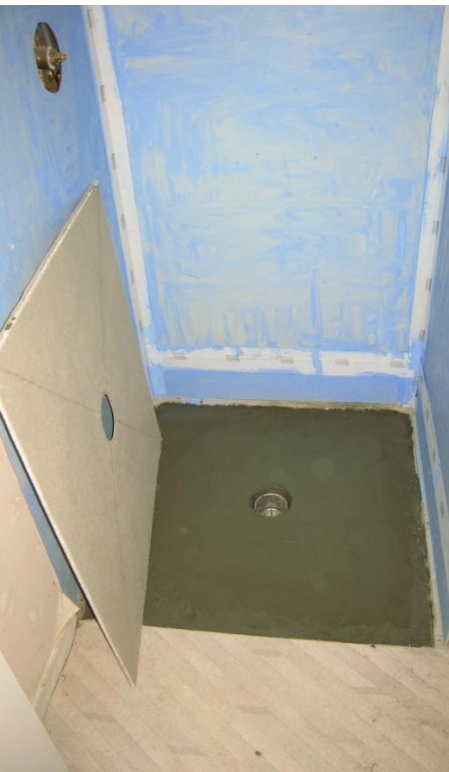
5. Waterproofing the walls & corners.
