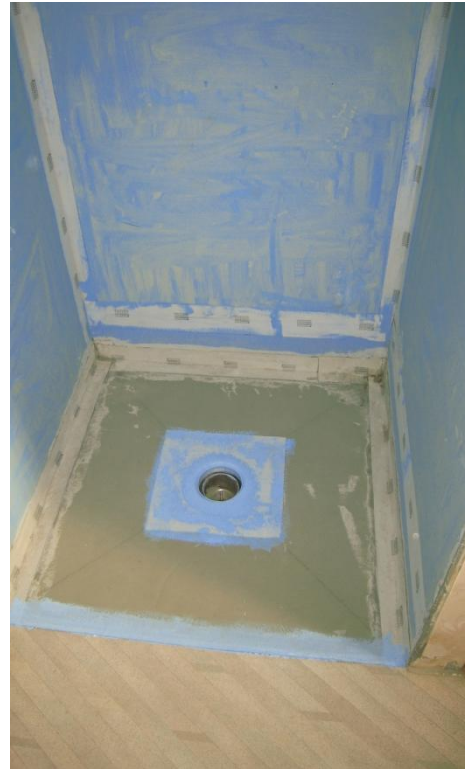
8. Waterproofing last corners & waste.
