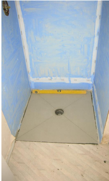
7. Leveling in the base.
