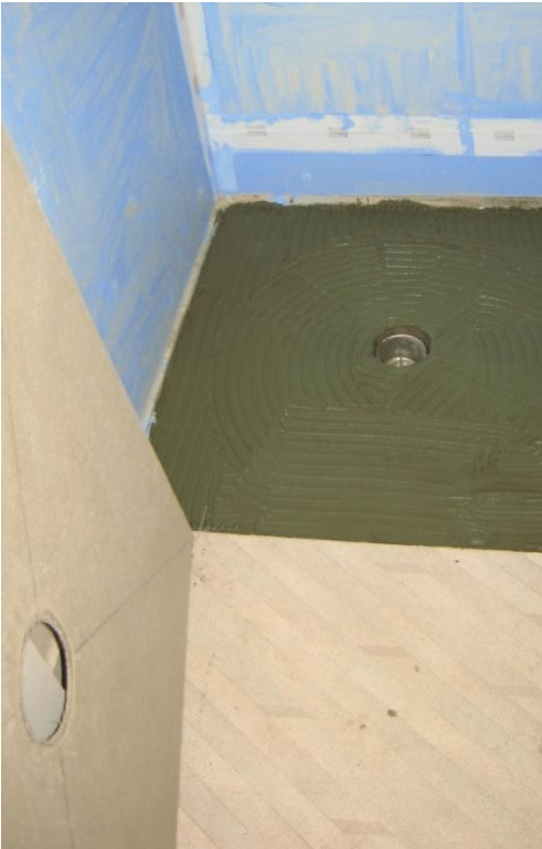
6. Fixing down the 10mm base.
