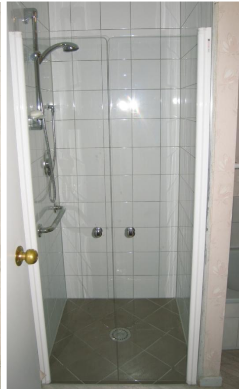
11. Finished step-in shower!
