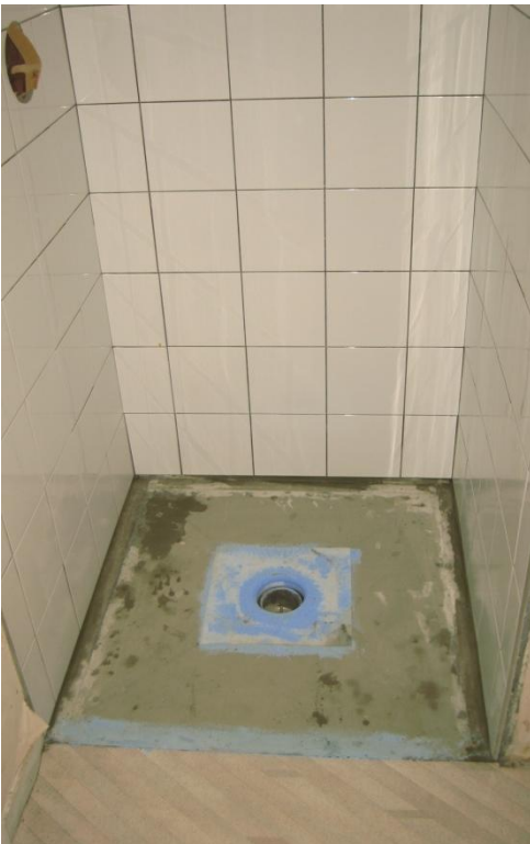
9. Tiling the walls first.
