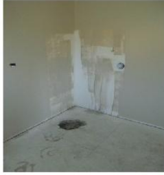
1. Breaking the concrete floor and find the waste pipe
