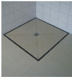
1. Finally get the base tiled and grate inserted
