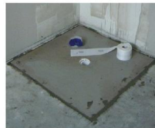
6. Installing and adjusting shower base
