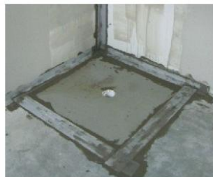
7. Sealing all corners and joints
