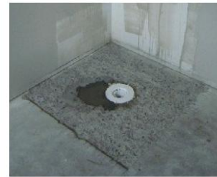
4. Connecting trap and shower drain to waste pipe
