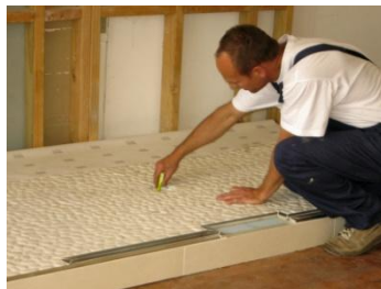
Carrying in the shower base and marking the hole for the drain pipe, drilling the hole, putting down the glue and positioning down the shower base
