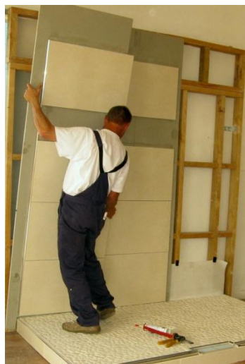
Fixing the wall panels to the studs by gluing and screwing. Using polyurethane glue and big head screws.
