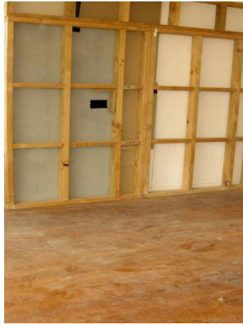
Typical situation at any bathroom.
