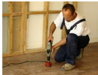
Carrying in the shower base and marking the hole for the drain pipe, drilling the hole, putting down the glue and positioning down the shower base
