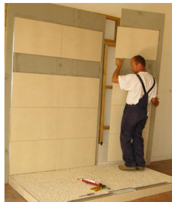
Fixing the wall panels to the studs by gluing and screwing. Using polyurethane glue and big head screws.
