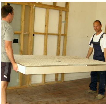
Carrying in the shower base and marking the hole for the drain pipe, drilling the hole, putting down the glue and positioning down the shower base
