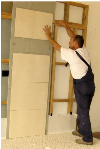
Fixing the wall panels to the studs by gluing and screwing. Using polyurethane glue and big head screws.
