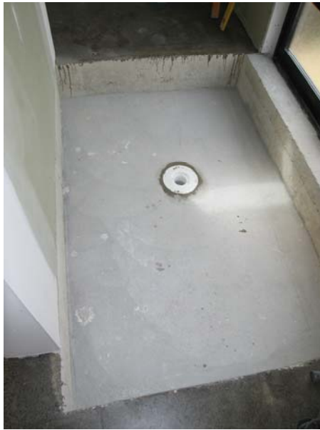
installing the leak control flange
