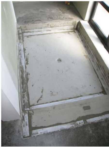
creating little step with 100 mm building board... sealing all corners with corner pieces and tape
