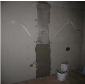
after reinforcing all joints panel can be plastered or tiled over...
