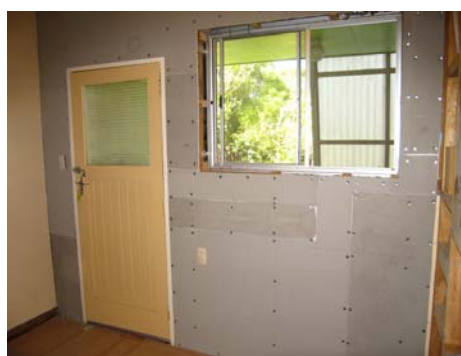
after reinforcing all joints panel can be plastered or tiled over...
