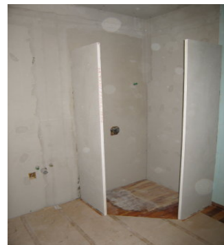
can be used as wall liners, either directly on timber studs or on top of existing linings
