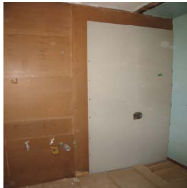
can be used as wall liners, either directly on timber studs or on top of existing linings
