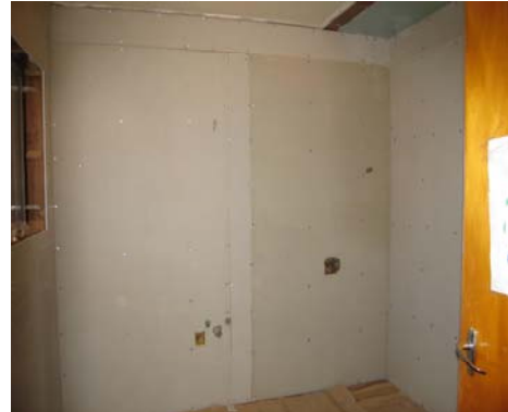
can be used as wall liners, either directly on timber studs or on top of existing linings
